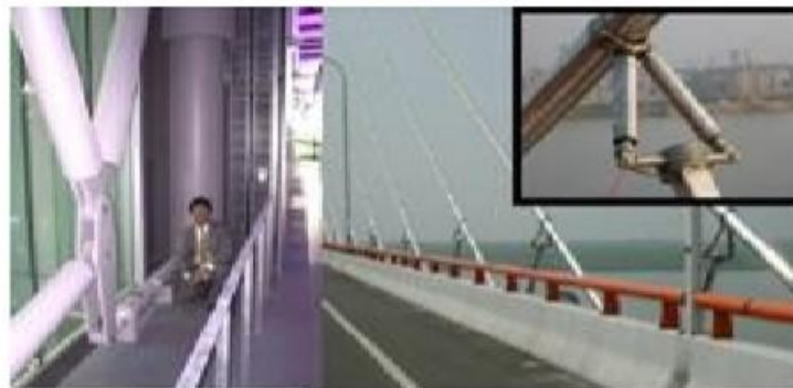
FIG. 9. Danting lake bridge – China [15]
