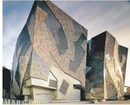
Fig. 26. Fractal applications on façade (Amal Osama, Fractal geometry in architecture: from formative idea to superficial skin design, 2014)
