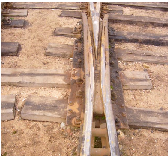
Fig. 3.8. Railway crossing assembly
