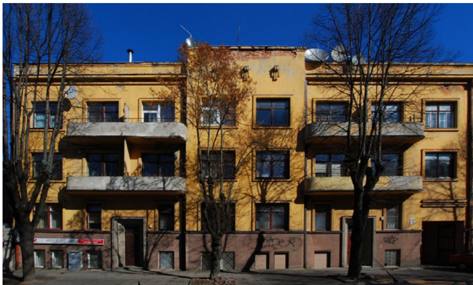
Fig. 3. The building at Miško Street, 16, which was demonstrated in the experiment
