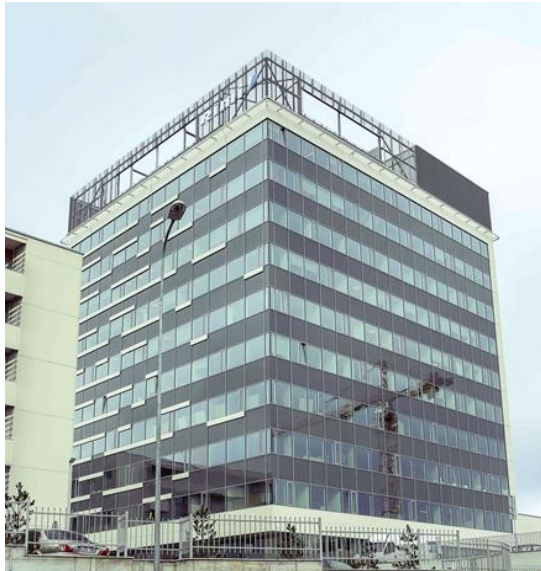
Figure 1 Photo of the building
