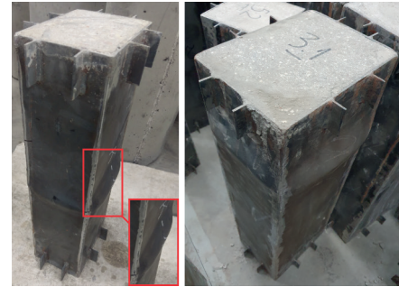
Fig. 3 Local buckling of the columns
