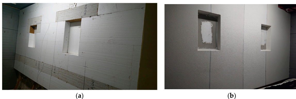
Figure 1. (a) EPS thermal insulation with mineral wool fire barriers; (b) test rig with 4 types of plastering.
