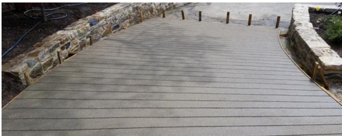
Figure 7. Lip or curb at sides of ramp reduces the risk of slipping off (Northshore, 2018).
