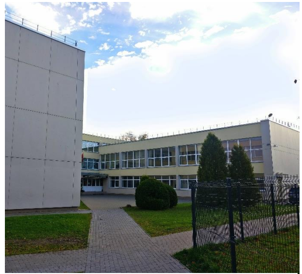
Figure 70. Site B – Renovated gymnasium.
