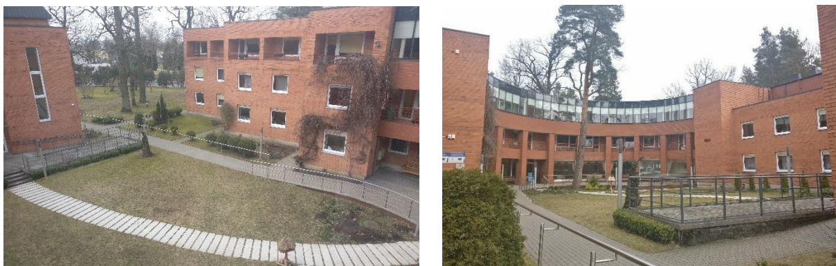
Figure 24. Kaunas Panemunė retirement home, courtyard.
