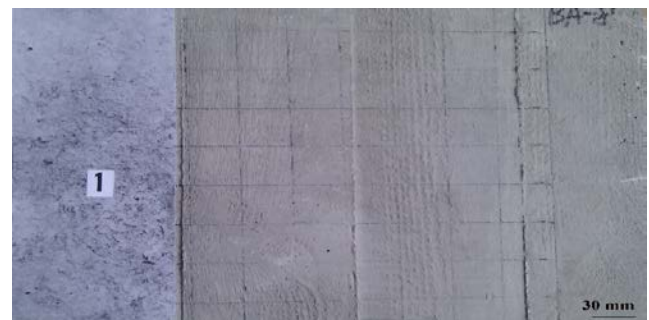
Fig. 5. Specimen's, taken from the sawn timber formwork, surface evaluation process (BA8 concrete mixture)
