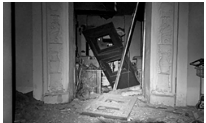
Fig. 24. Photo of the destruction inside the architectural monument – Kharkiv Airport VIP terminal [17].
