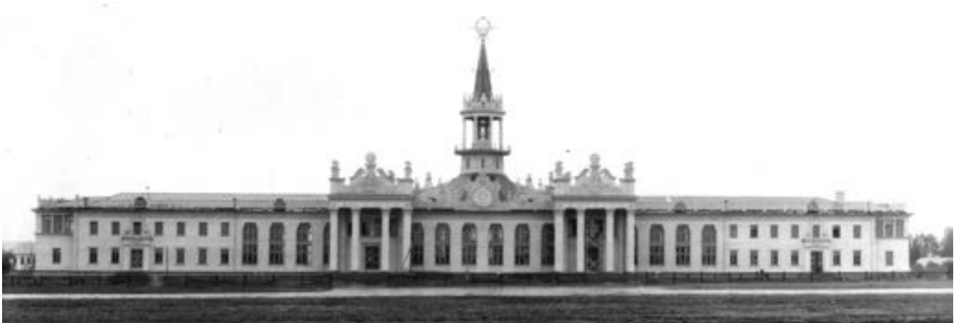
Fig. 3. Kharkiv Airport terminal, the facade facing the airfield, 1954. [Photo from the private archive of A. Saratov].
