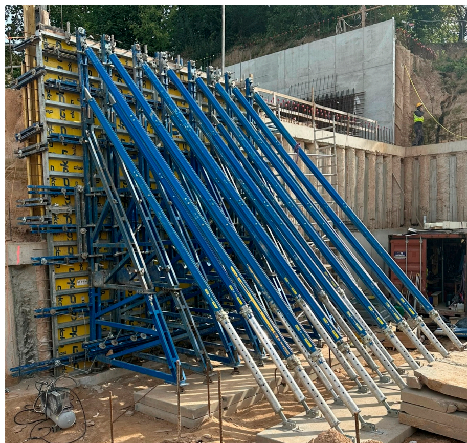
Figure 1. View of the formwork setup on site.
