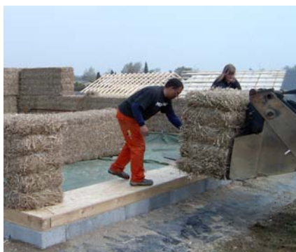
Fig. 7. Construction using big bales, Denmark. Photo by Lars Keller
