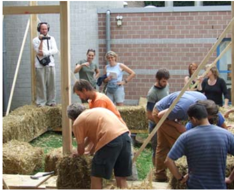
Fig. 4. Load bearing construction, Belgium. Photo by Edita Milutiene
