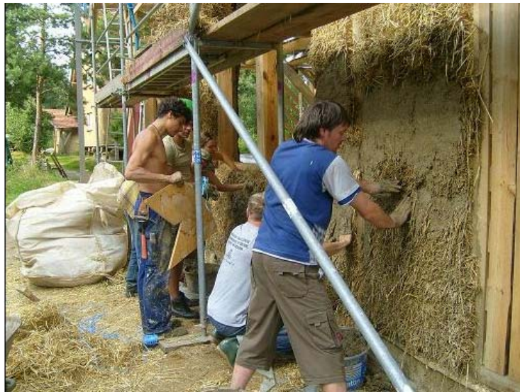
Fig. 3. Straw bale house under construction. Photo by Arturas Gobys
