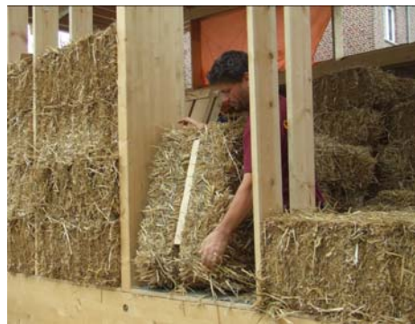
Fig. 5. Frame construction, Belgium. Photo by Edita Milutiene
