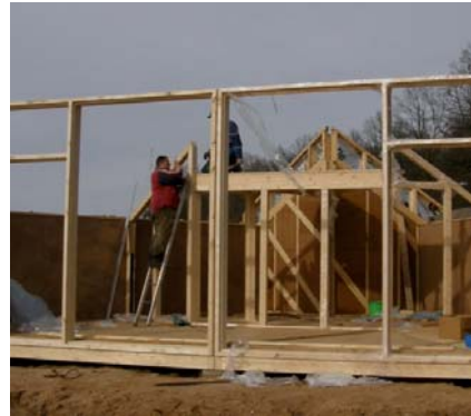
Fig. 6. Panel construction, Lithuania. Photo by JSK Ecococon
