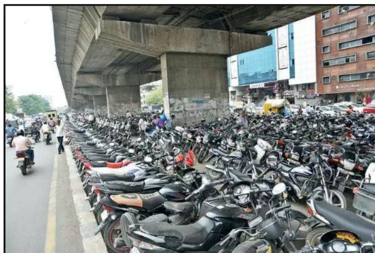
Figure 3. Flyover as a source of parking space
