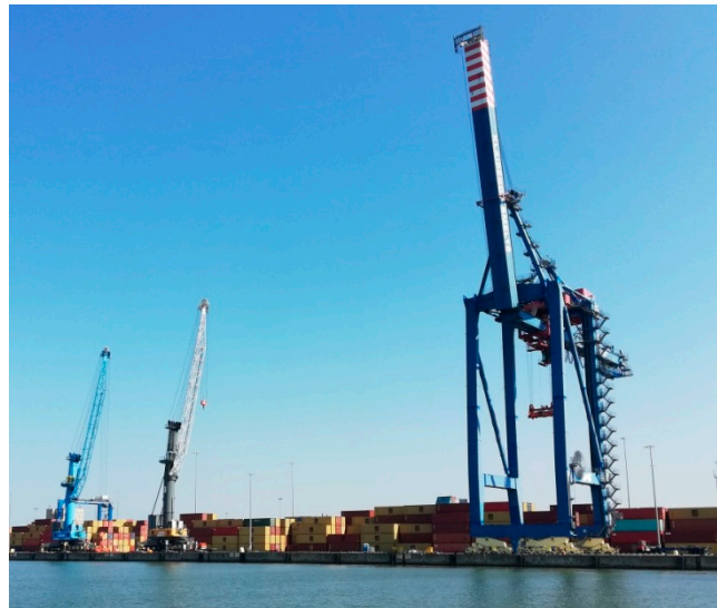
Figure 2. Container loading using one STS crane and one or two mobile cranes.
