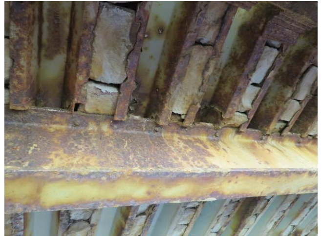
Fig.20 Bottom middle stringer and beams
