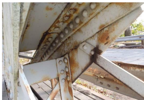
Fig.24 Broken connection upper first support
