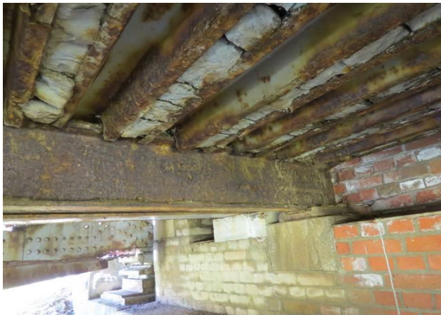
Fig.21 Bottom end stringer and beam significant corrosion
