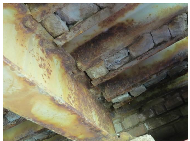
Fig.19 Bottom stringer significant corrosion
