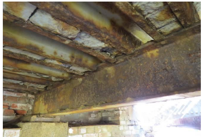
Fig.21 Bottom end stringer and beam significant corrosion
