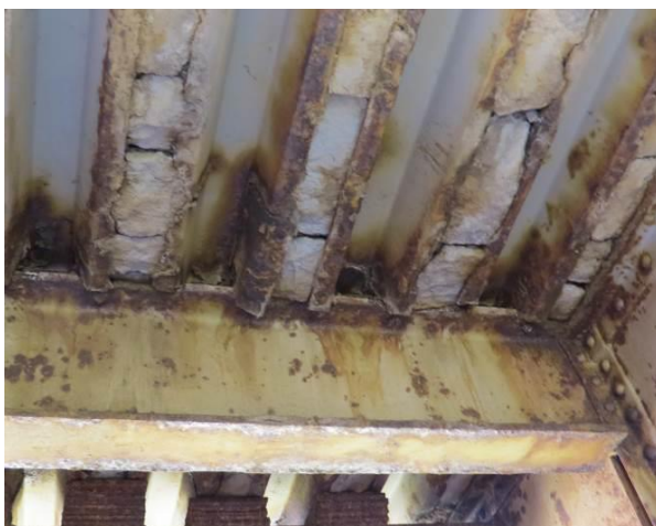
Fig.19 Bottom stringer significant corrosion
