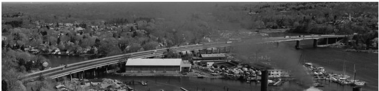
Fig. 2 Mianus River Bridge on Interstate 95 in Connecticut
