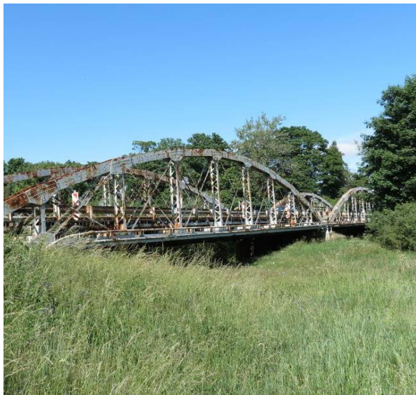
Fig.15 Bridge up stream
