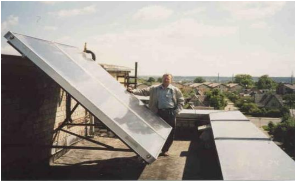
Solar collector of the DHWS system on the roof of Lithuanian Energy Institute
