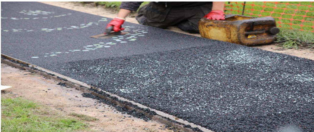
Fig. 28. Glow stones manual installation on Asphalt Road [Source: Photo retrieved from http://www.imagine7.co.uk/glowstones/ ]
