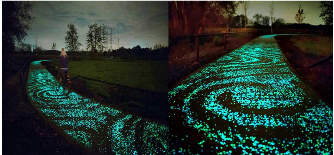
Fig. 20. Luminescent Aggregate Concrete Road [Sources: Core Glow Product Gallery, Retrieved from http://www.coregravel.ca/products/core-glow/ ]
