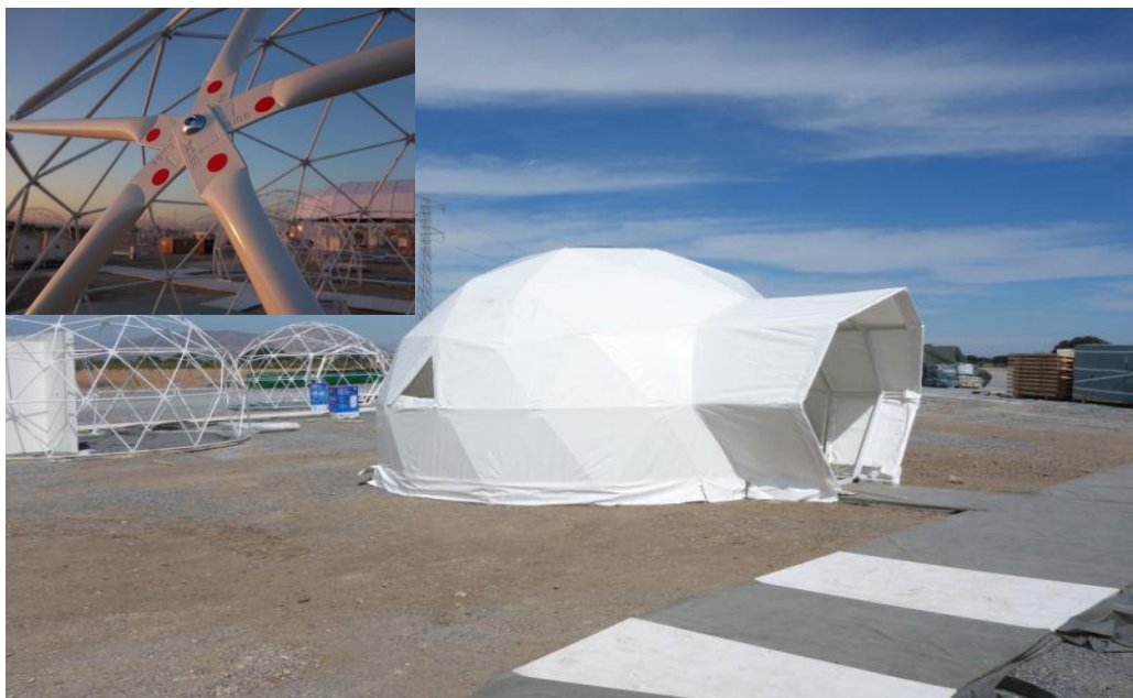
Fig. 25. Flattened Conduit Dome Structure in Sierra Nevada, Spain [Source: Photo retrieved from http://www.xcube-engineering.com/projects/glamping.html ]
