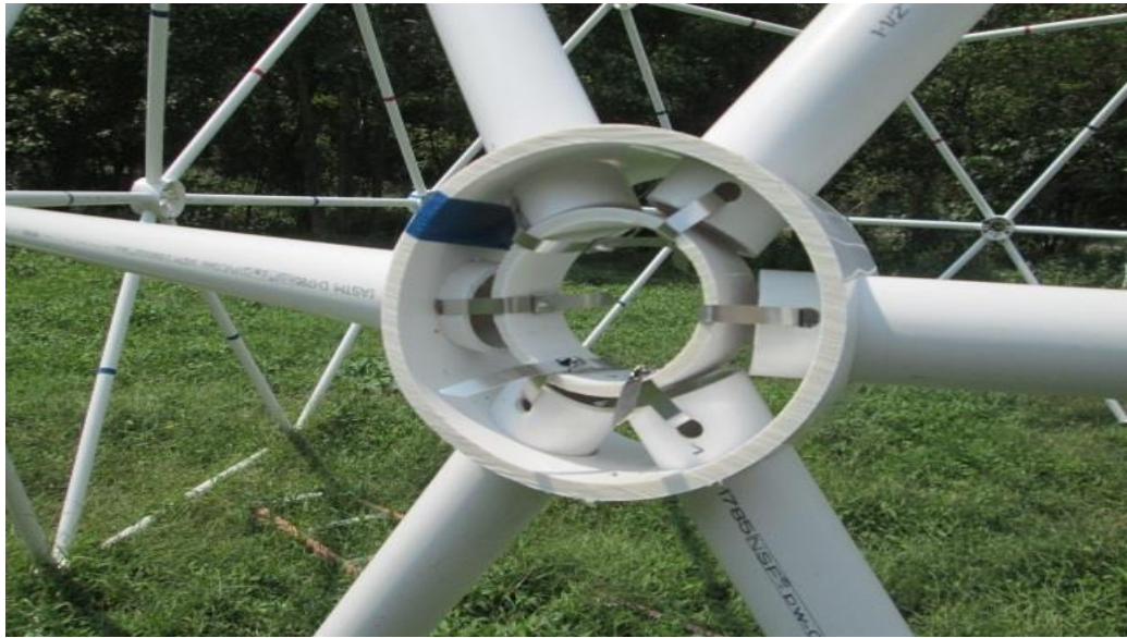
Fig. 26. Tube and Hub Jointed Dome Structure [Source: Photo retrieved from https://www.ziptiedomes.com/geodesic-shelter-domes/index.htm ]
