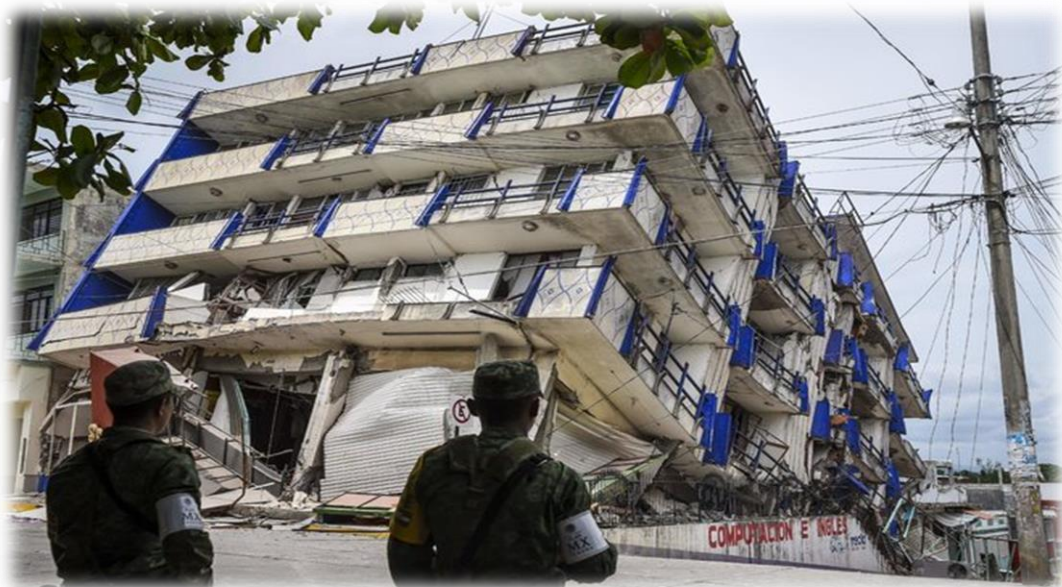
Figure 4 The Photograph shows a row the 4 story Building collapsed due to 8.1 Magnitude.
