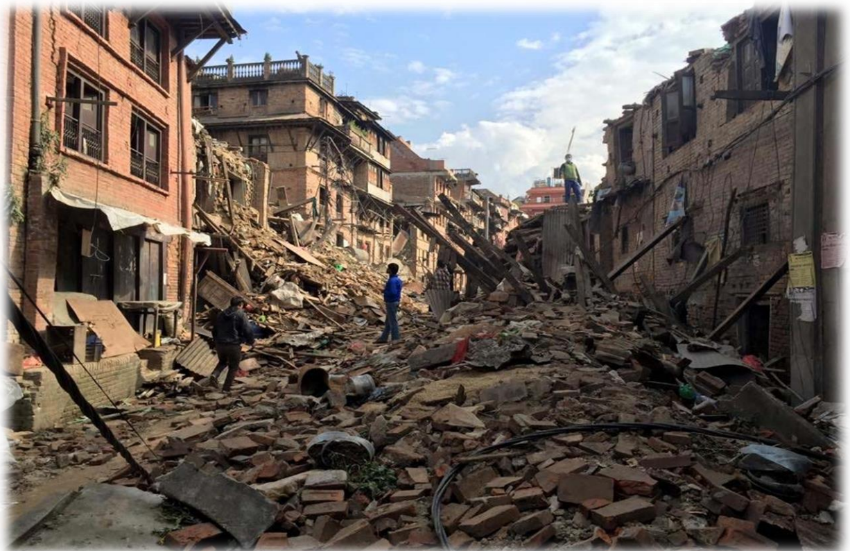
Figure 2 : “This building shows how it damaged the adjacent building due to earthquake, P.C: Matthew Wood.”
