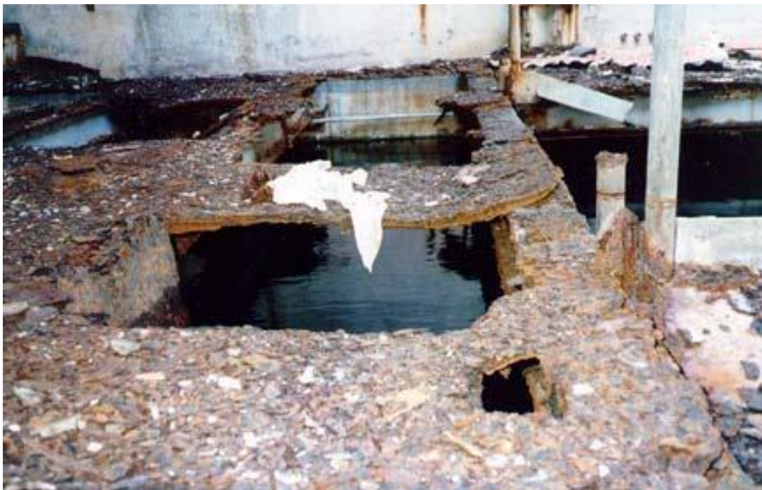
Fig. 1.1 Corrosion process on metal [1]
