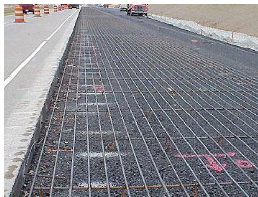
Figure 3 Schematic Presentation of steel reinforcement constructed on S.R. 288 in Virginia
