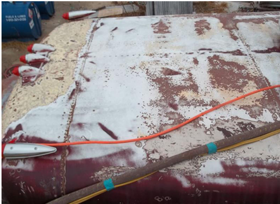
Fig. 3.1 Surface before blasting
