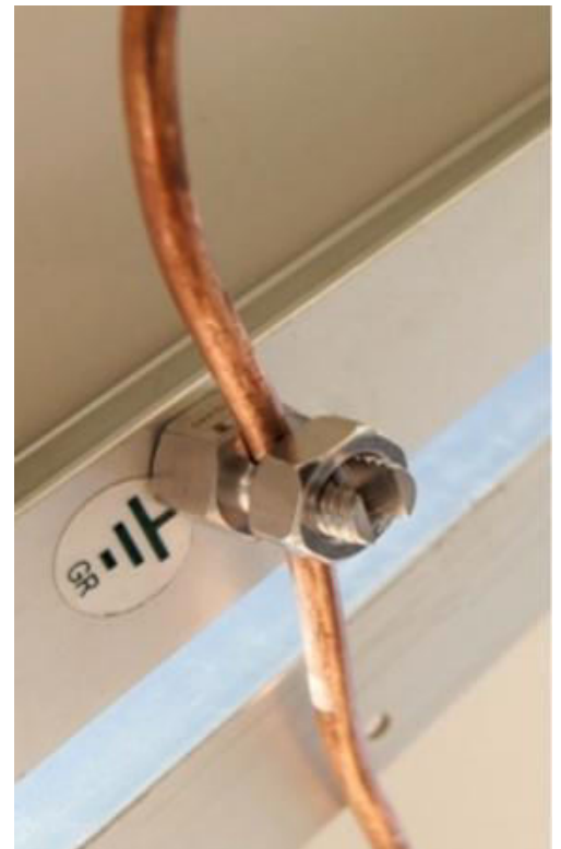
fig.. 5.7 circuit connected to ground
