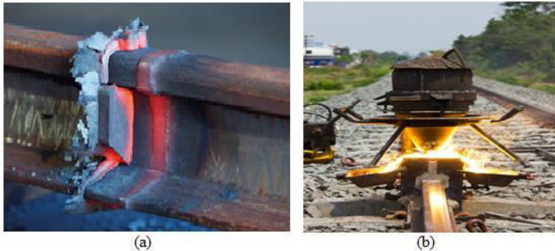
Fig.1.4. (a) Flash butt weld [8] (b) Alumino-Thermic (AT) Weld [9]
