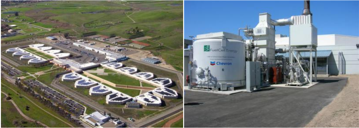
Figure 3.4 Example of Microgrid at "SANTA RITA JAIL - CALIFORNIA" [49]
