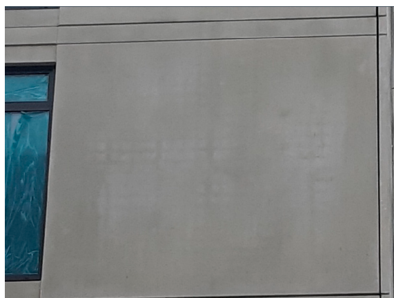
(a) Precast concrete wall
