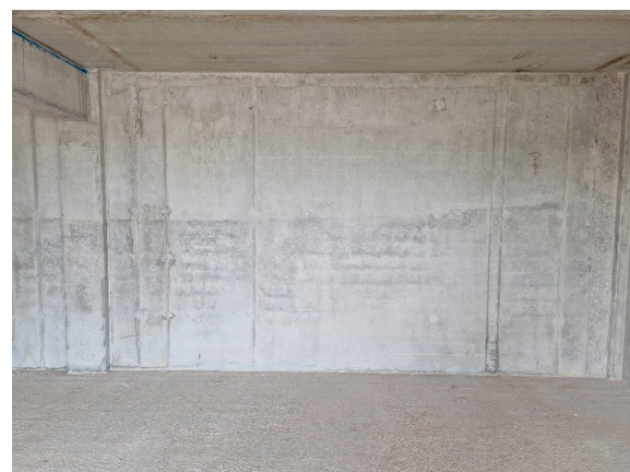
(b) In situ cast concrete wall
