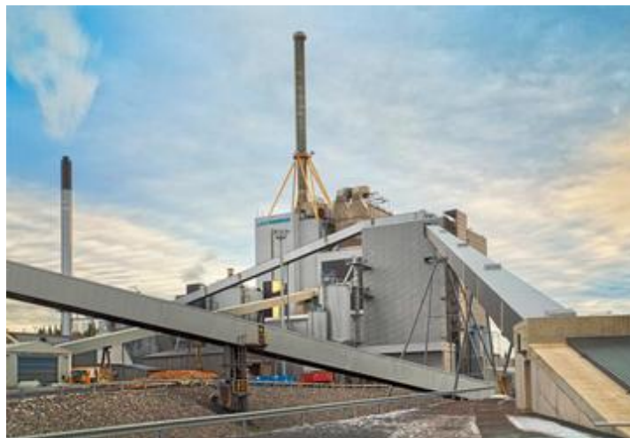
Figure 2.2. Lahti Energy's power plant
