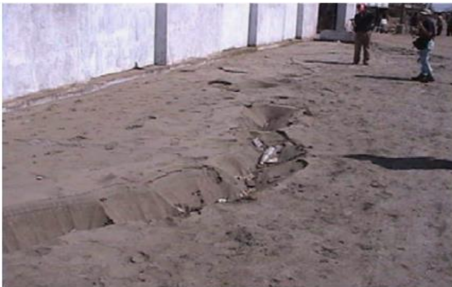
Figure 7 Deposition of liquefied sand through ground cracks Bhuj earthquake 2001 India(EERI archives)
