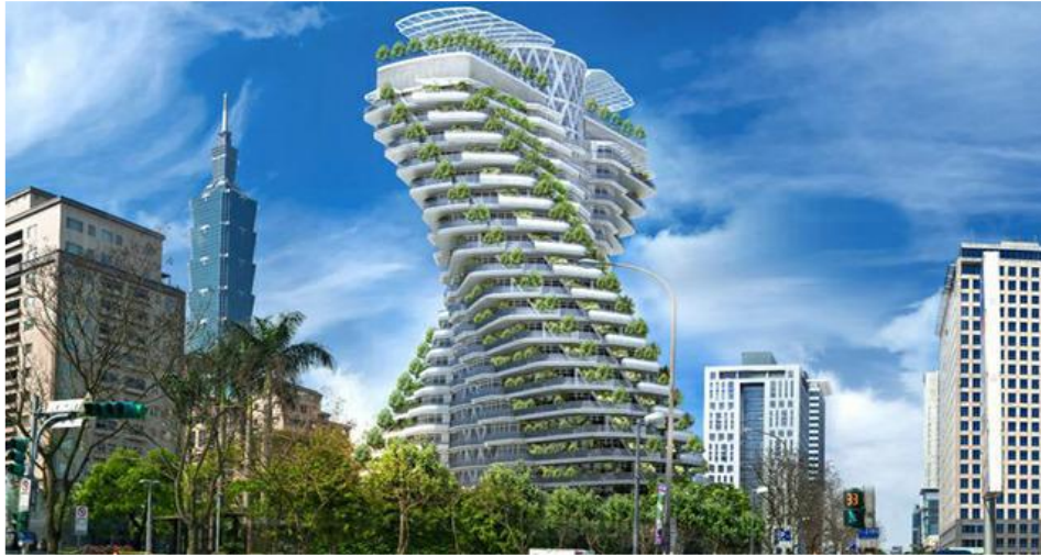
Figure.3. Agora Garden tower. Downside view.
