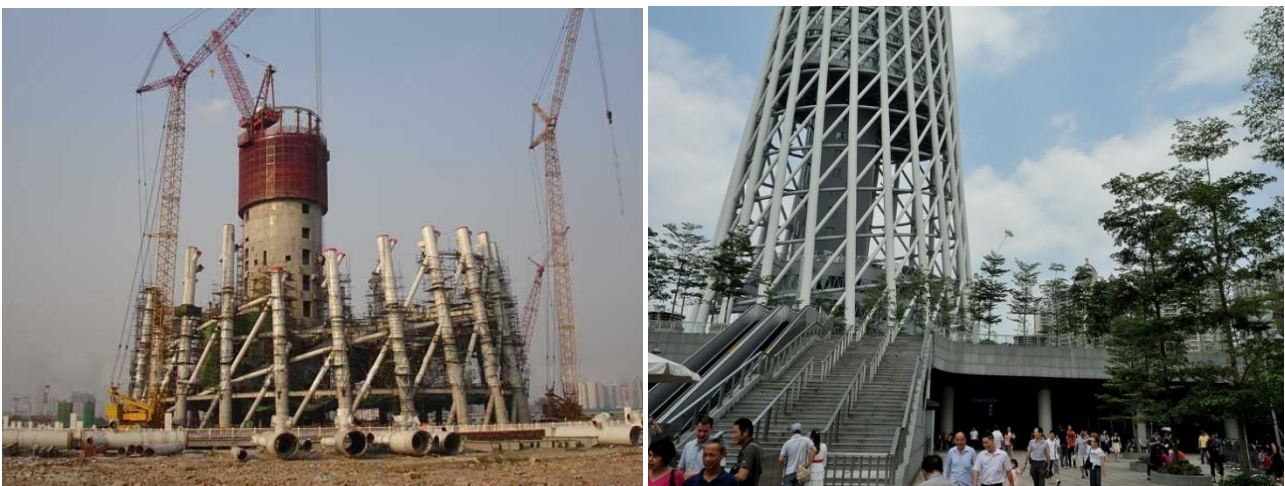
Figure.4. Canton tower. Construct view and downstairs position view.
