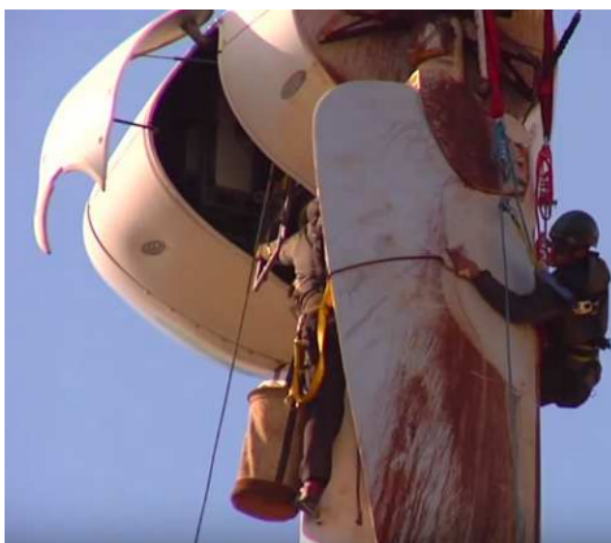
Figure 1. Manual cleaning of wind turbine blades.
