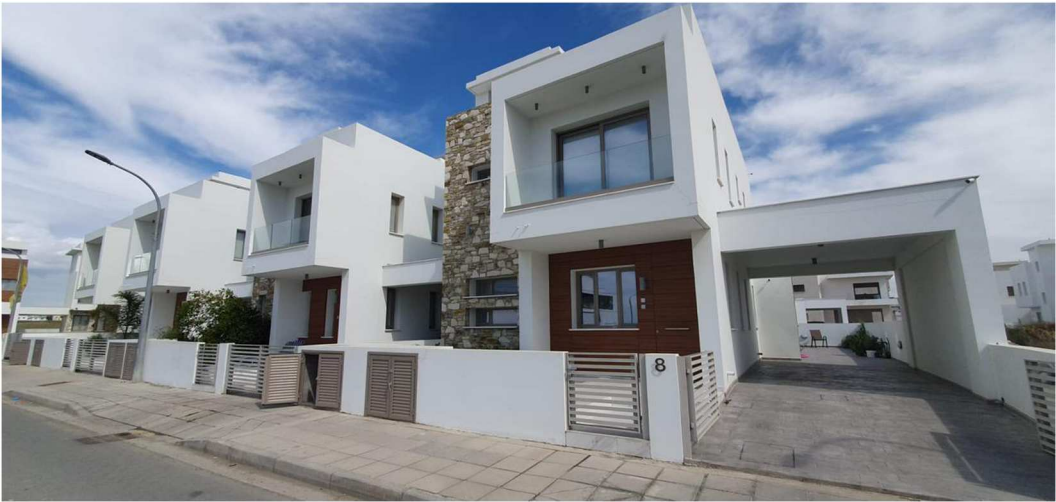
Figure 1. Examined complex of buildings.
