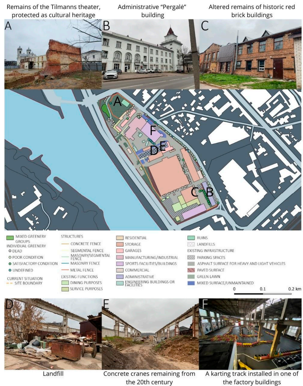
Figure 4. Present-state analysis scheme and view of current ruins site and its buildings. The letters on the map identify the objects and spaces recoded in the photographs. Photographs and scheme by D. Zmejauskaitė.
