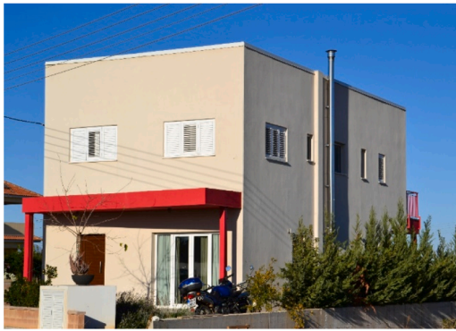
Fig. 4. Exterior view of pilot building in Nicosia, Cyprus.
