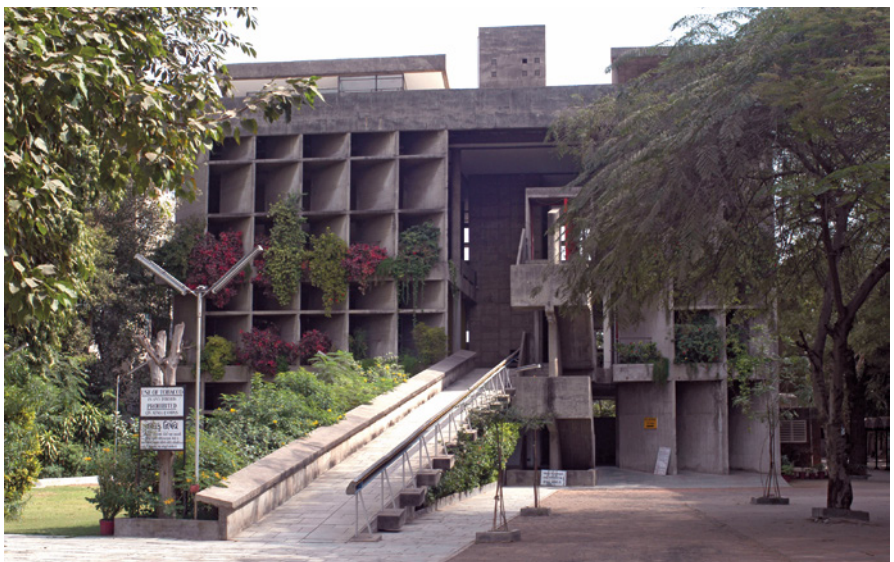
Figure 131 View of the front garden and ramp at the Mill Owners' Association, Ahmedabad. © Jan Haenraets, 2005.
