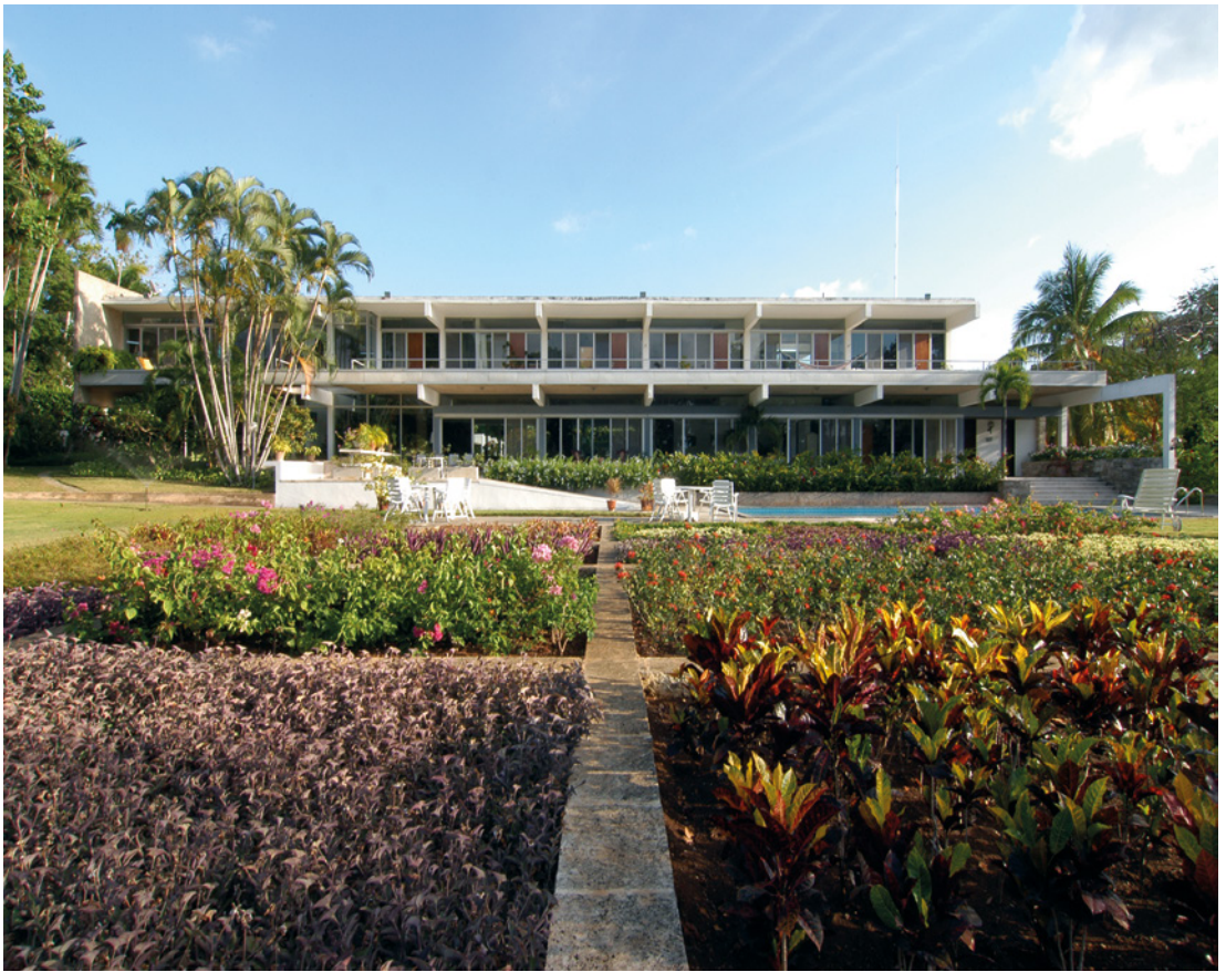
Figure 21 View from the Garden of the De Schulthess Residence towards the house. © Eduardo Luis Rodríguez Archive, 2006.
