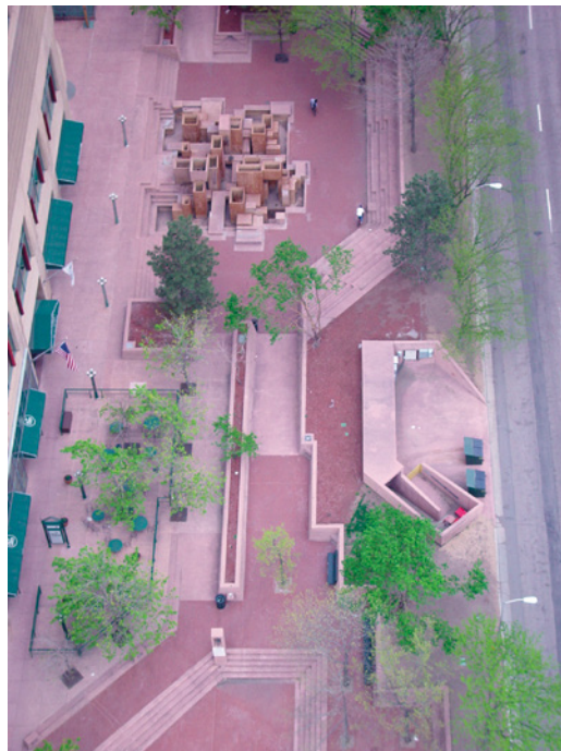
Figure 103 View eastward from the D&F Tower, showing the second block between the Sixteenth Street Mall and Seventeenth Street, with the plaza area below the tower, a service area centre to the right, and the signature fountain. © Ann Komara, 2003.
