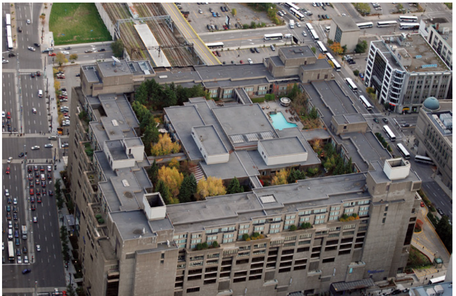
Figure 89 Aerial view of the rooftop garden. © Hotel Bonaventure Montréal.
