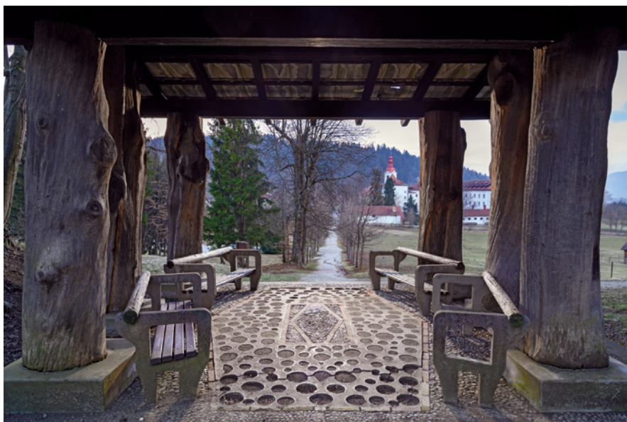
Figure 171 The wooden pavilion, with paving in stone, exposed concrete, brick, wooden cuts, and benches of Murka Brezjanka, designed by Jože Plečnik, with the view towards the chestnut promenade. The promenade leads to Begunje church and the castle, which serves as a psychiatric hospital with the park used by patients and the public. © Miran Kambič, 2021.
