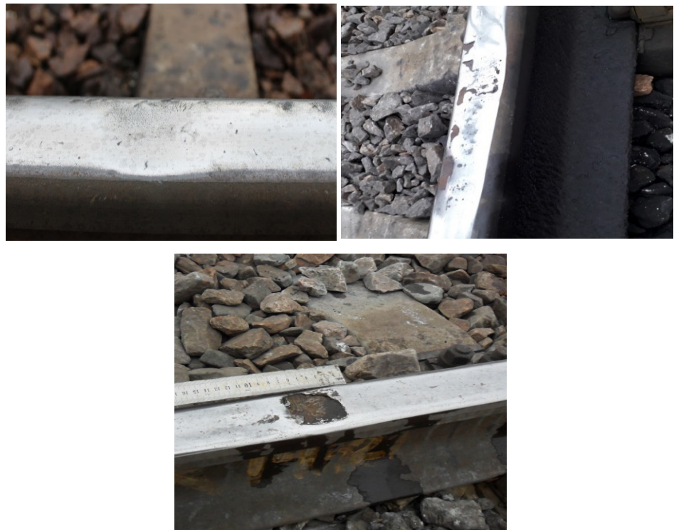
Figure 2. Types of controllable surface rail defects (photographs taken by the authors).
