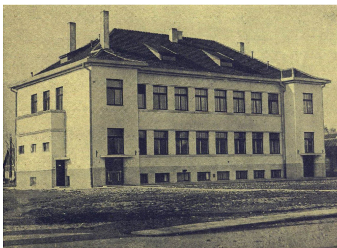
Fig. 5. Administrative building of Trakai County Municipality in Kaišiadorys (civ. eng. Pranas Rudys, 1933) [photo from Savivaldybė, No. 2, 1940, cover page ].
