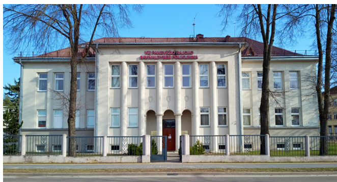
Fig. 6. Former administrative building of Panevėžys County Municipality (civ. eng. Petras Lelis, 1939) [photo by author, 2024].
