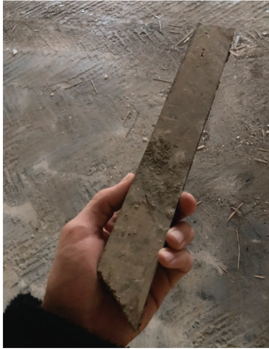
Fig.3 REMAIN 3b, picture of a floor fragment, photograph by Breg Horemans on November 8th 2022, courtesy of Breg Horemans. Detached piece of parquet, saved from demolition. The piece of wood has a tar layer on the bottom. The remain is saved as part of TAAAT's Live Archive.
