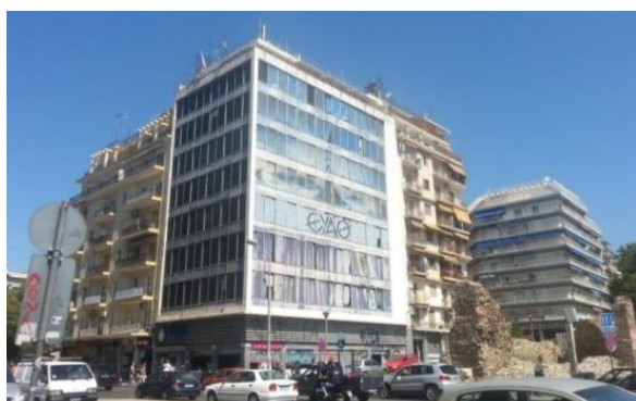
Figure 3. Exterior façade of the examined building.
