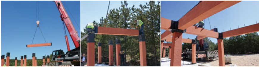
Fig. 14.8 Installation of beams
