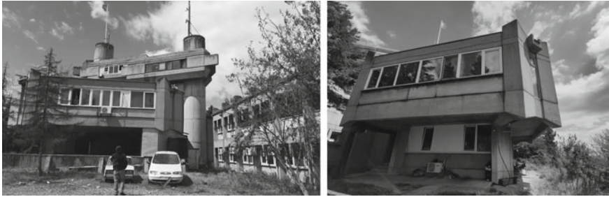
Fig. 34.1 Different views of Hydrometeorological Service building
