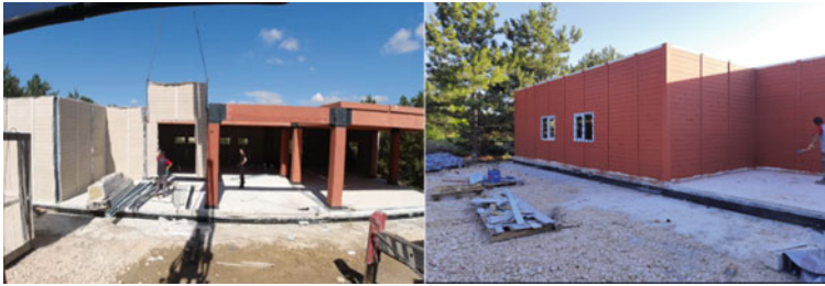
Fig. 14.10 Installation of non-structural elements
