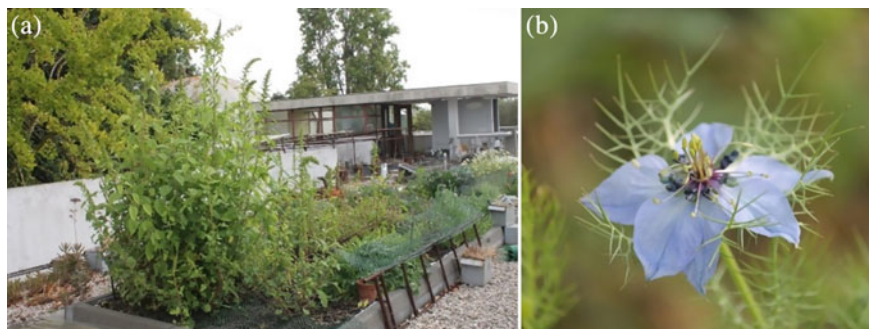
Fig. 28.4 a Green roof built at the Instituto Superior de Agronomia campus—as part of the green roof lab, Universidade de Lisboa, Portugal; b detail of Nigella damascena plant. Original images from Paço, T. A
