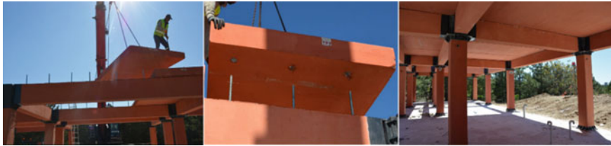
Fig. 14.9 Installation of slabs
