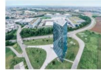
15 AutomationCenter | Germany | 2017 | DGNB | Platinum
