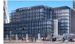
18 SKYSAWA Building A Poland | 2016 | BREEAM | outstanding
