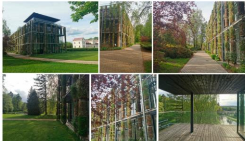
Figure 3. Vilnius University Kairenai Botanical Garden’s Green Building-Plant with external layer of vegetation was selected as an example of applied biophilic design. Photographs by A. Daugelaite.
