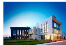
33 Smart Building Center-W.P.I.P Poland | 2016 | LEED | Platinum
