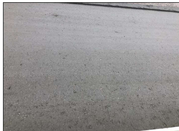
Fig. 54. RCC after running rubber tyre roller compactor machine
