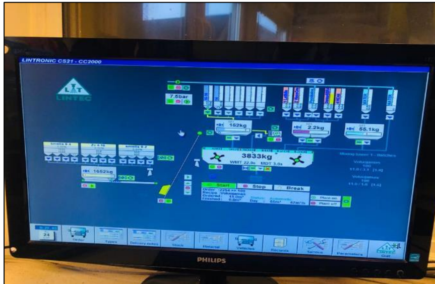
Fig. 47. Concrete batching plant system monitor
