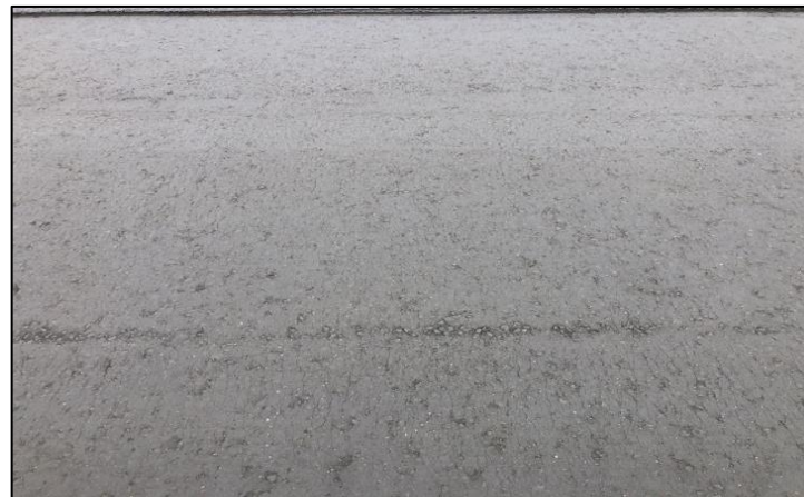
Fig. 54. RCC after running rubber tyre roller compactor machine
