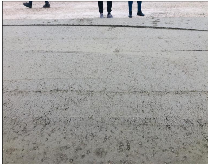
Fig. 53. RCC after running roller compactor machine
