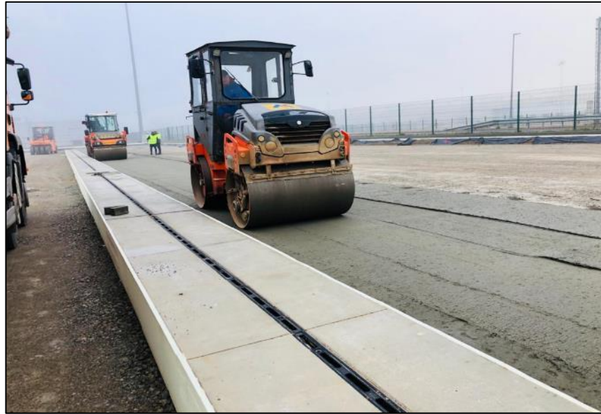
Fig. 51. RCC Roller compactor machine
