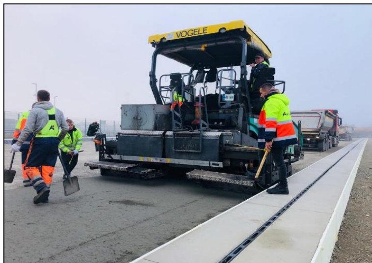
Fig. 50. RCC Paver machine
