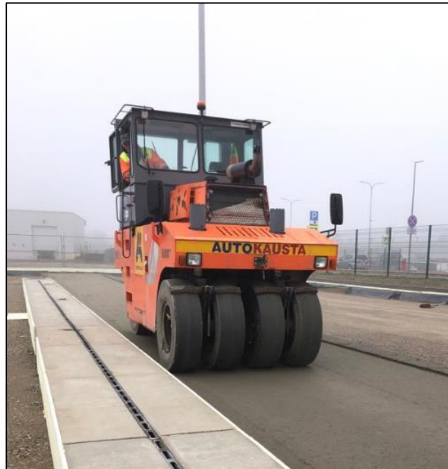
Fig. 52. RCC Rubber tyre roller compactor machine
