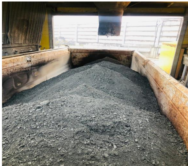
Fig. 48. RCC dumped in truck
