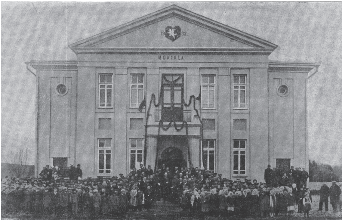
Fig. 2. Primary school building built in the early 1930s in the small town of Aukštadvaris based on the standard design developed in 1925 at the request of the Ministry of Education. "Tautos mokykla" 1 (1933), cover page
