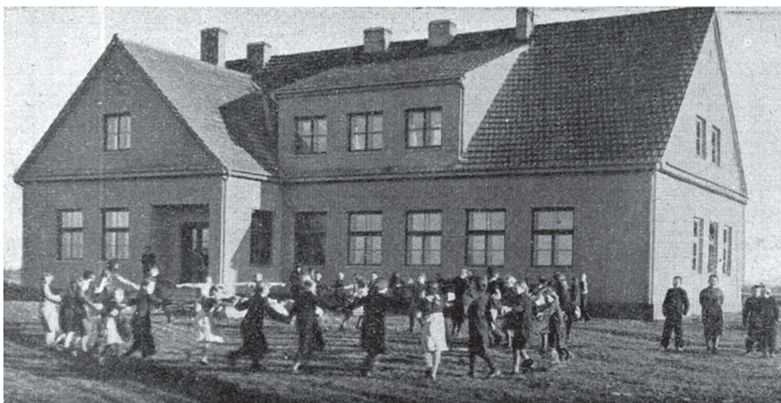
Fig. 10. Masonry primary school building built in the mid-1930s in the village of Rėkliai based on the recommended standard design developed from award-winning design submitted to the architectural competition held in 1936 by the Ministry of Education. "Tautos mokykla" 24 (1938), 563
