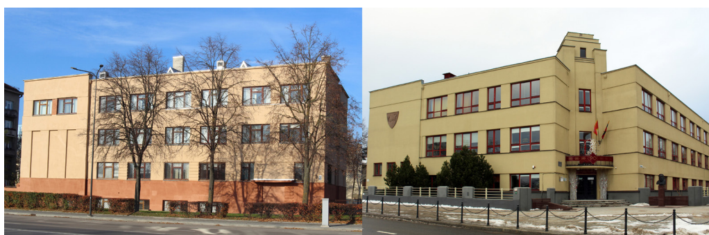
Fig. 4. Former primary school buildings in Kaunas (civ. eng. Antanas Jokimas, 1930) [photos by author, 2022].
