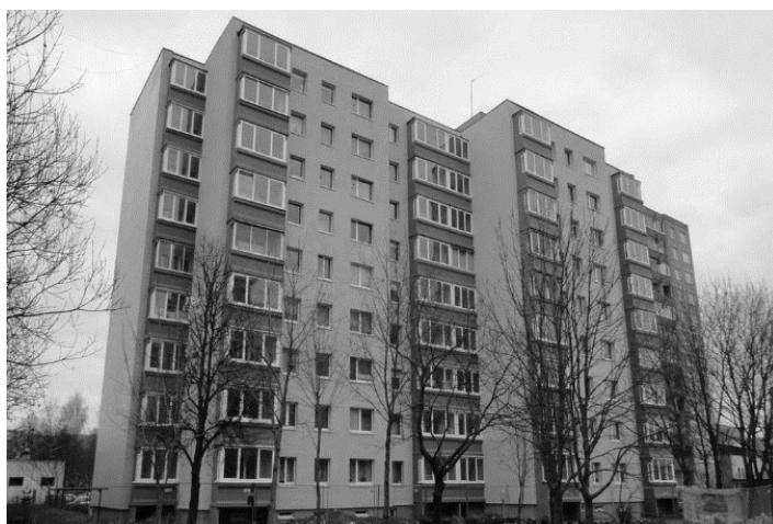
Fig. 5. Renovated multi-apartment building (Building A)
