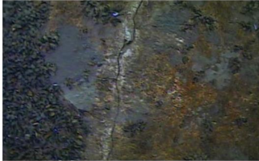
3 fig. An example of an optical image of underwater crack on the dam surface (taken from [40])
