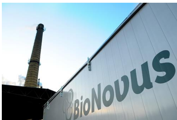
Fig. 1.1 “First Opportunity” boiler house [1]
