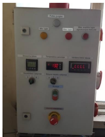
Fig. 5.4 Water temperature under pressure test
