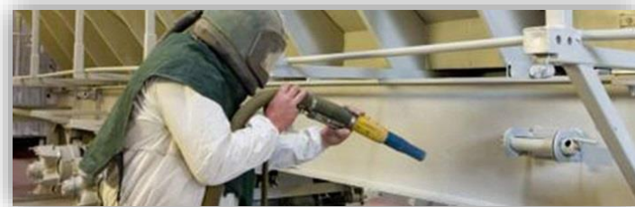
Fig. 1.3 Surface cleaning with abrasive blast [2]
