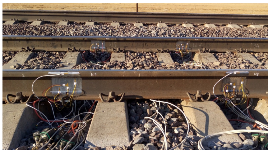
Figure 5. Sensor layout (photograph taken by the authors).
