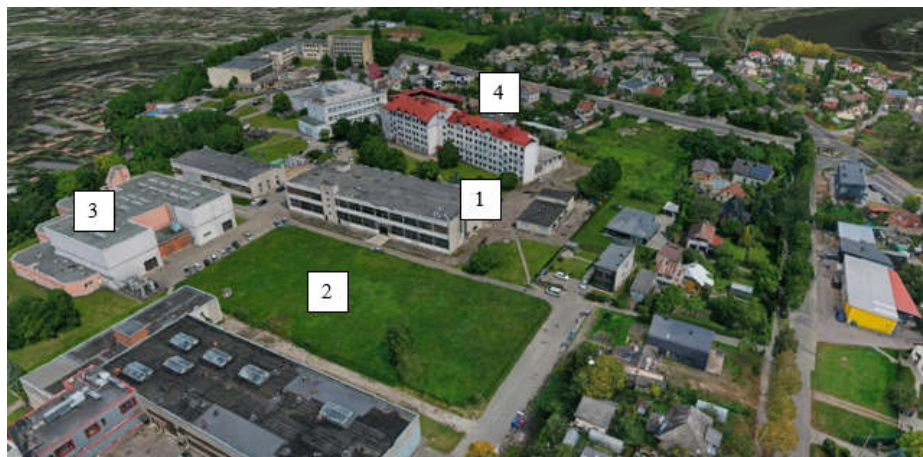
Figure 1. PV module locations: 1—flat roof, 2—ground, 3—south wall, and 4—pitched roof.
