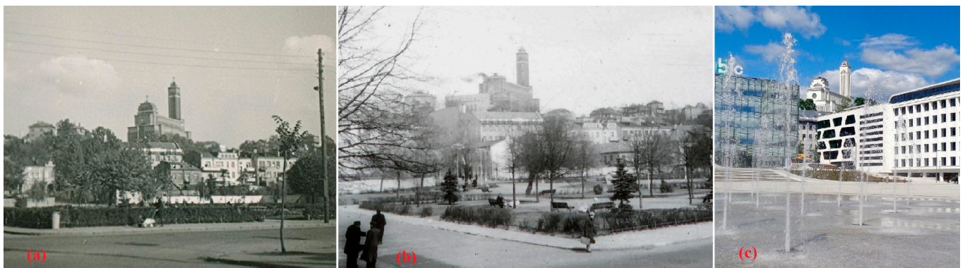
Figure 7. Christ’s Resurrection Church. View from the city’s lower terrace. (a) 1930s (source: Kaunas City Museum); (b) 1960s (photographer Stanislovas Lukošius, source: Kaunas City Museum); (c) 2020 (photo courtesy of Arvydas Pakštalis).
