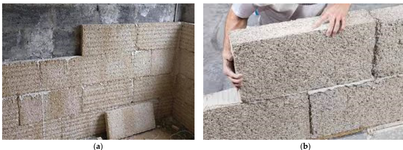
Figure 3. Example of (a) hemp blocs and (b) positioning of hemp concrete (reproduced from [33]).
